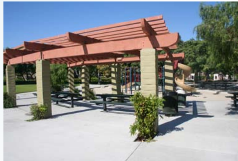
Shadowridge Park Pavilion
